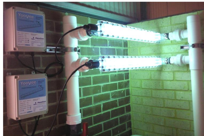
Twin Manifold Chloramine Removal 100,000 litres
